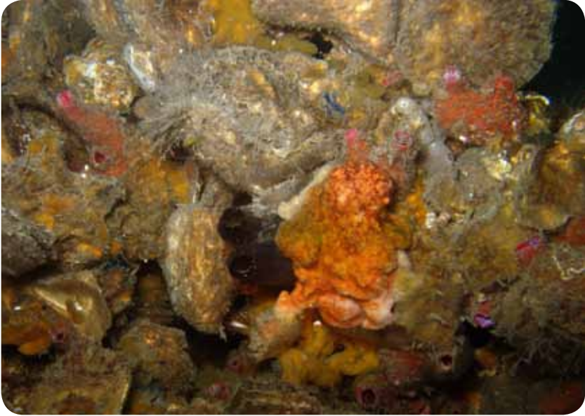
Figure 43: Oysters ( Ostrea edulis ) are the major bioconstructors of the fouling community formed on the pier-columns in the Port of Koper.
