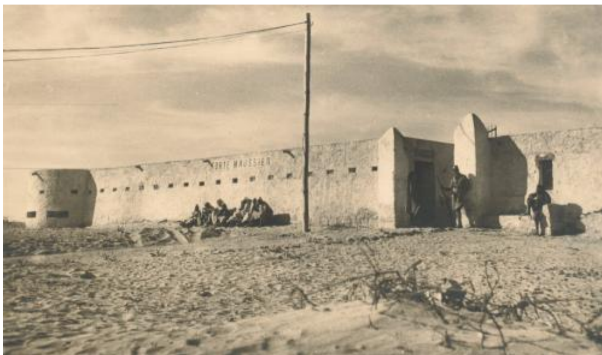
Figure 1 : Saffron Palace. (Photo. © General Authority for Culture (Sirte Office))
