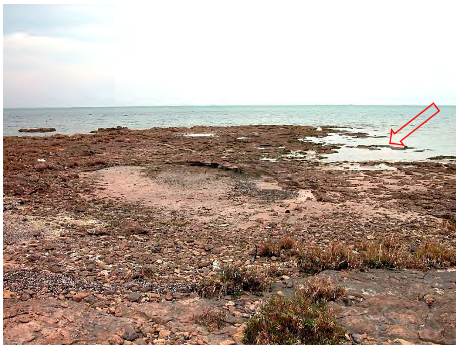
Fig. 15. Corroded sandstone veneer with signs of erosion (arrow)
