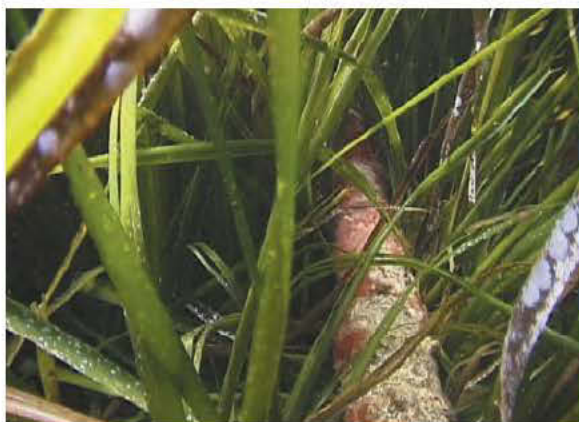
Fig. 113. The electric cable between Corsica and Sardinia, simply laid over the meadow near Cala di Sciumara (Corsica). 35 years after it was laid (in 1967) there is no negative impact on the meadow. From Pergent et al. (2002b).
