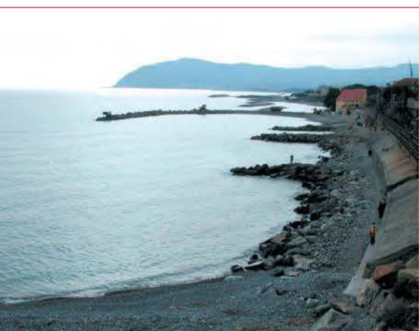
Fig. 63. Cervo (Imperia province) facility for defence against erosion of the coast and the railway line (Settore Ecosistema Costiero archives – Liguria region).
