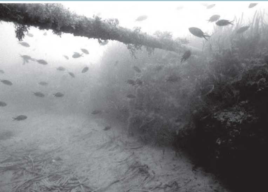
Fig. 108. An underwater cable, exposed and precariously balanced, in Marseille (Prado Bay). The erosion scarp in the Posidonia oceanica meadow is visible on the right. From Charbonnel et al. , 1999). Photo by E. Charbonnel.
