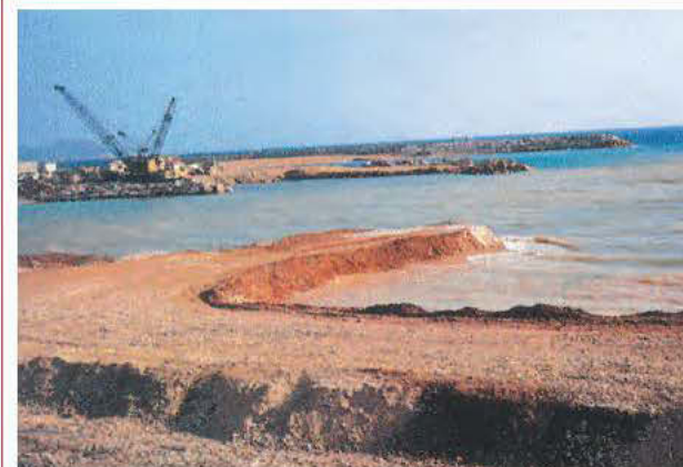
Fig. 59. Developing Le Mourillon's artificial beaches (Toulon, Var, France). Fine sediment is carried off by hydrodynamism. From Astier et al. (1980).
